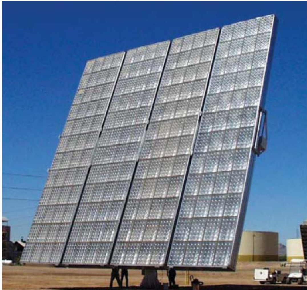
A concentrator system using Fresnel lenses (Amonix)
