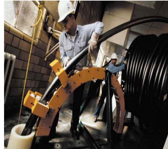
Detroit Edison cable installation (Courtesy, Pirelli)
