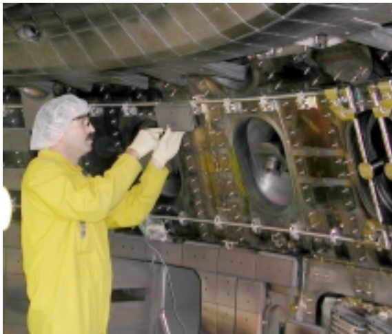
Fig. 1. Control coils (long rectangular objects) being installed in DIII-D.
