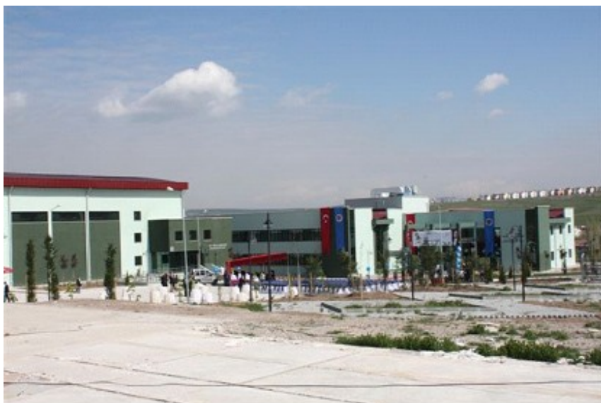
The opening ceremony of the first buildings of the Accelerator Technologies Institute, and the IR-FEL building, May 9, 2011, Gölbaşı, Ankara, Turkey.
