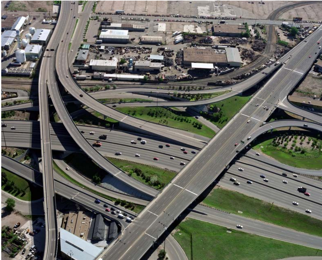
Photo: Warren Gretz/NREL
