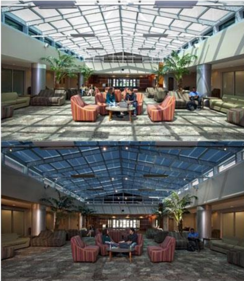
Smart Windows" seen at light and dark settings. | Photo Courtesy of SAGE Electrochromics, Inc., by Susan Fleck Photography
